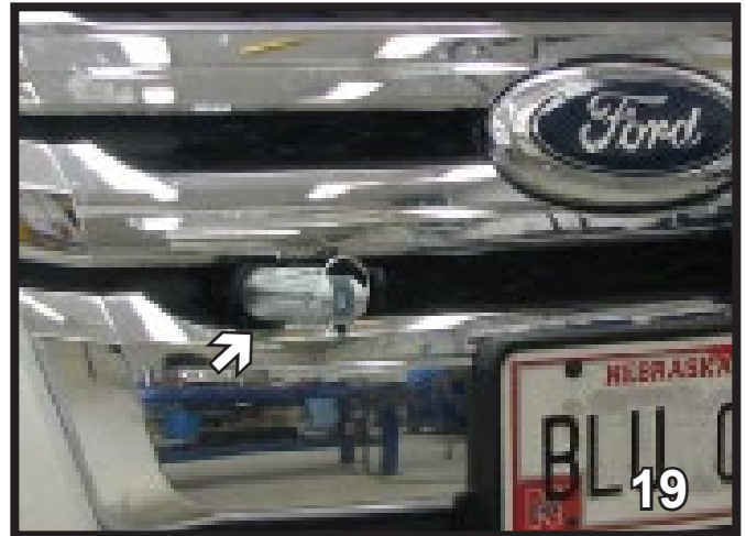
19. Align the fascia to its original position and using a utility knife, trim grille area in front of the attachment tabs. This will then create an opening for the tabs to come through, when reinstalling the fascia. Do this to both sides of the vehicle.
